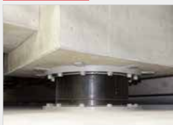
Figure B.3.1 A Seismic Base Isolation System.
