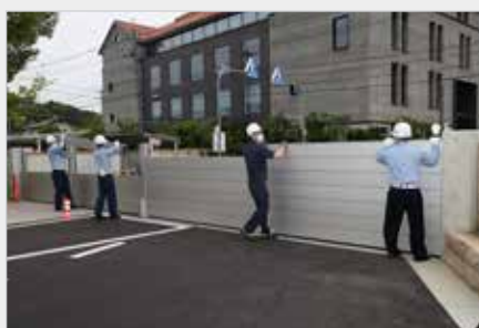
Figure B.4.1 Installation of Flood Barrier by Kurashiki Central Hospital Staff, June 2024.
